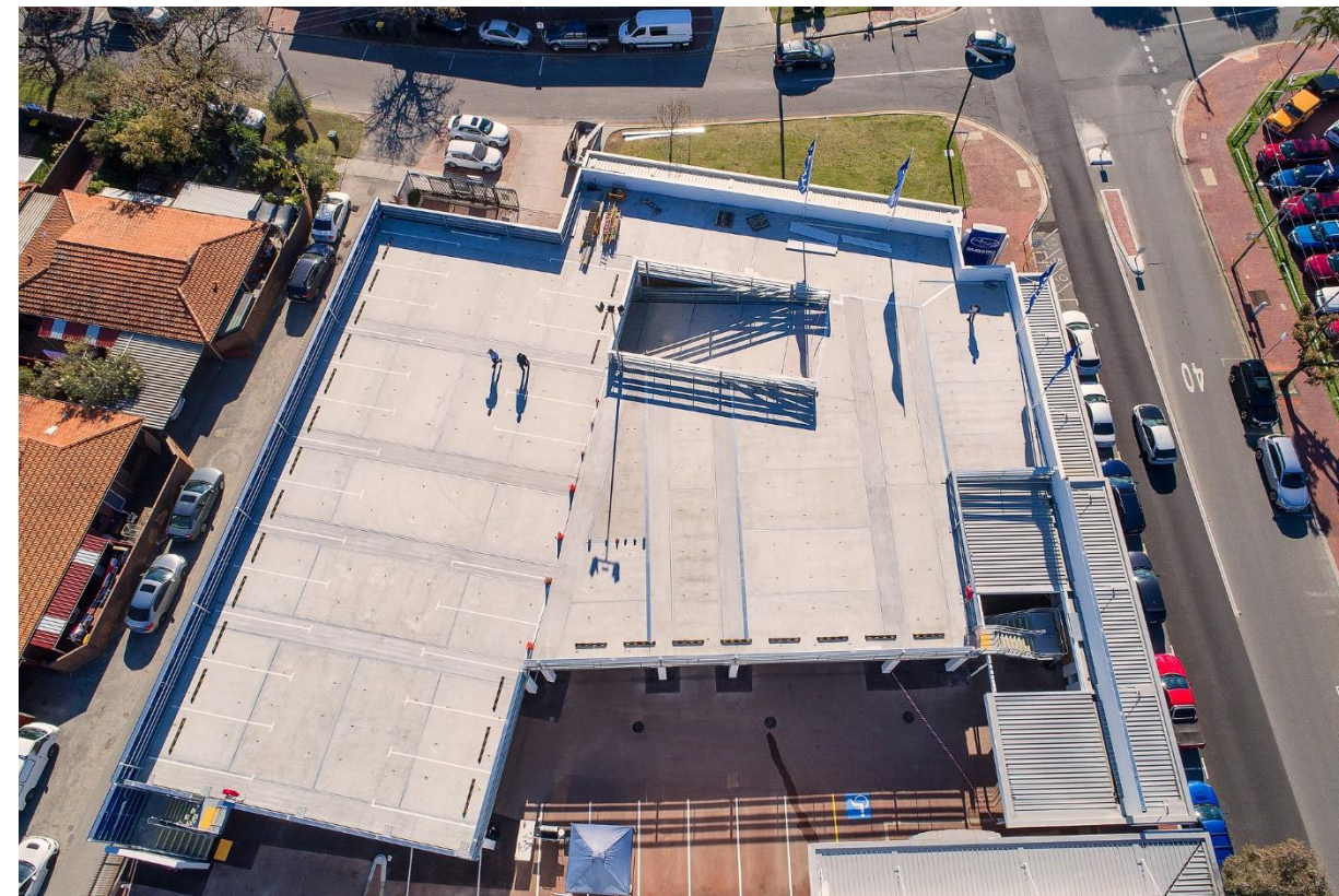
Crane Day 12. Substantial completion of structure
