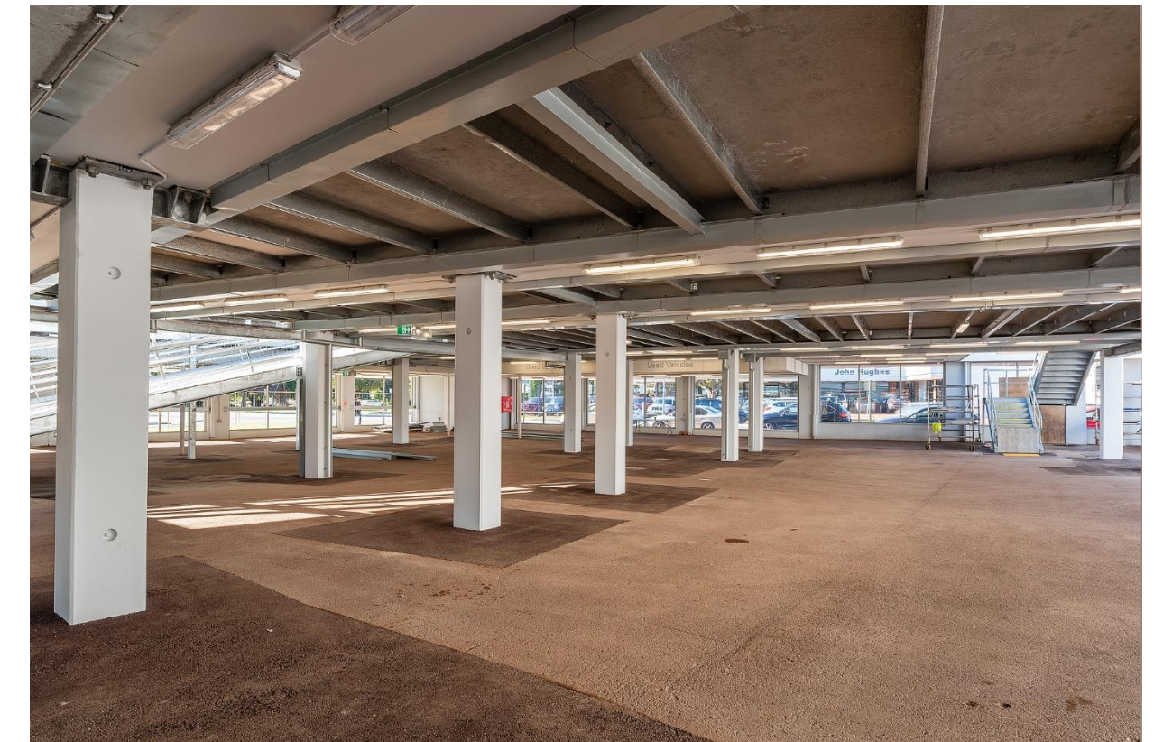
View of underside of the car park structure at Practical Completion
