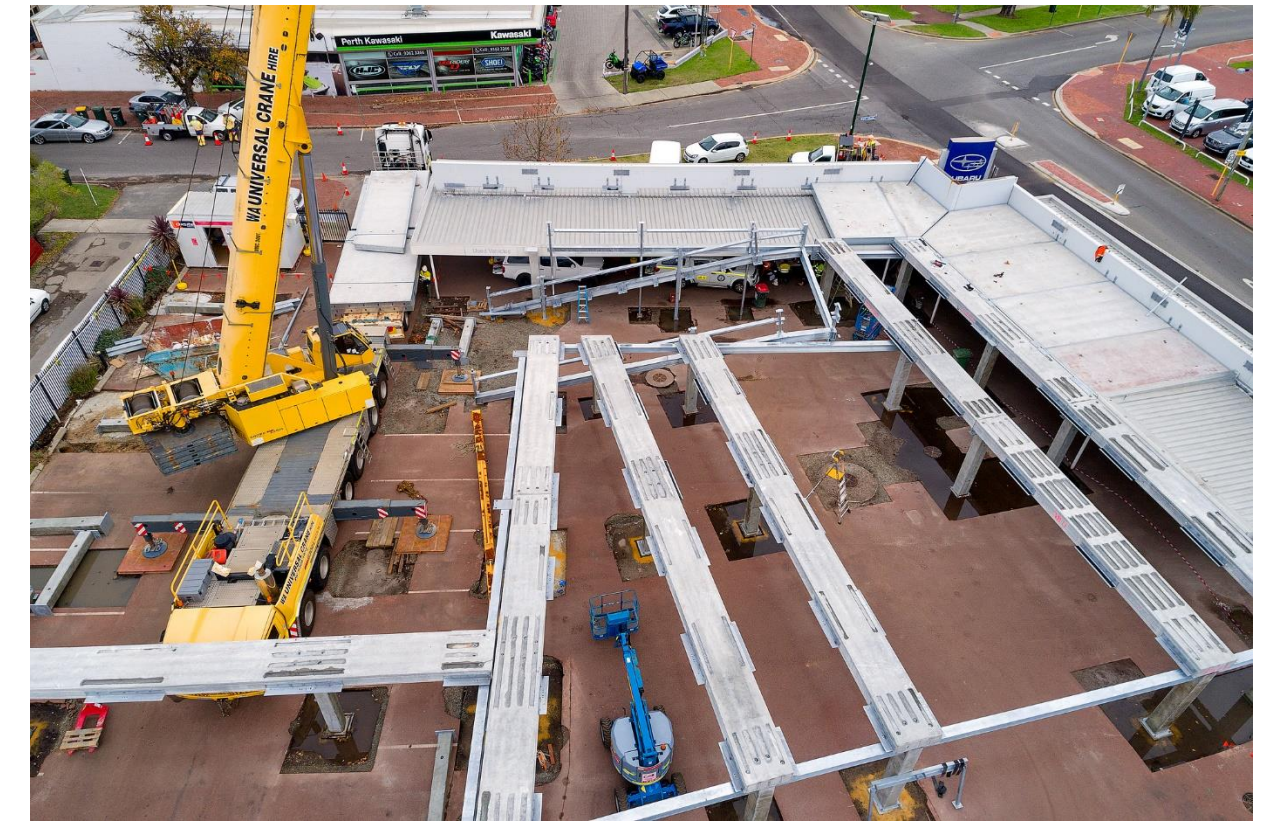
Crane Day 4. Slab panel installation
