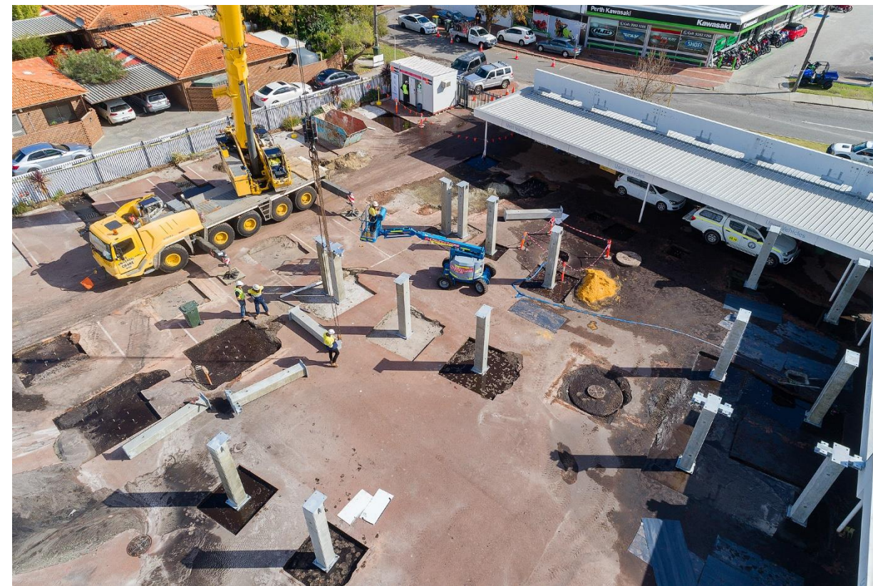
Crane Day 1. Column installation
