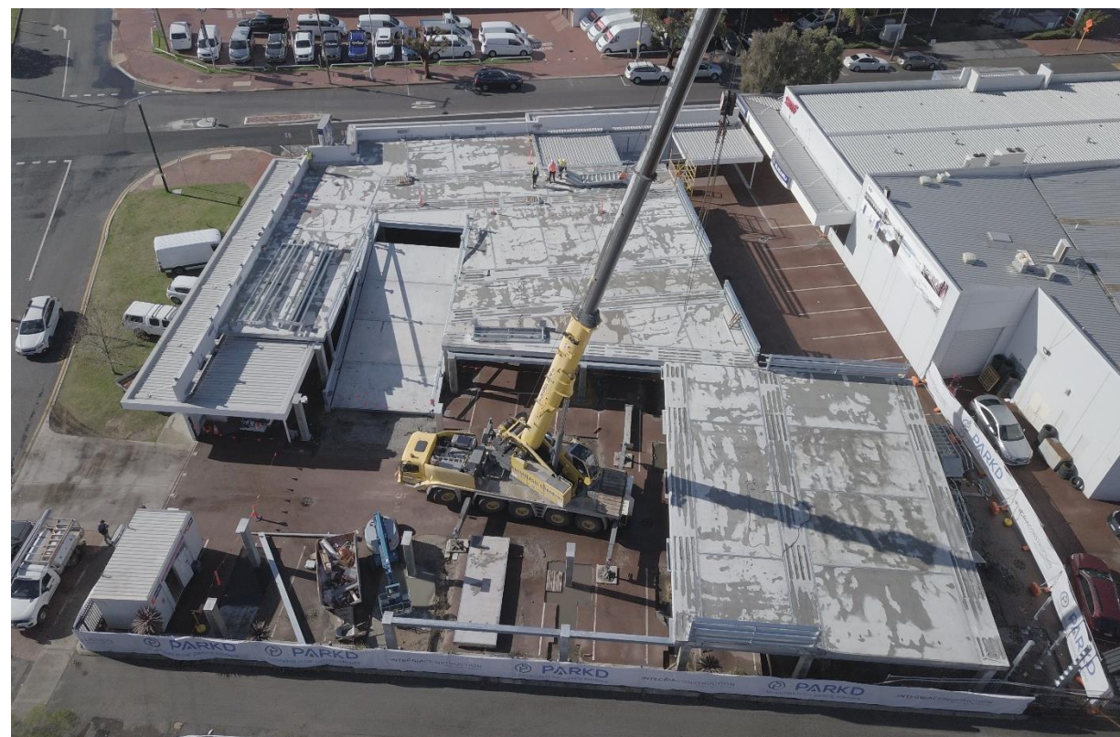
Crane Day 6. Slab panel installation complete
