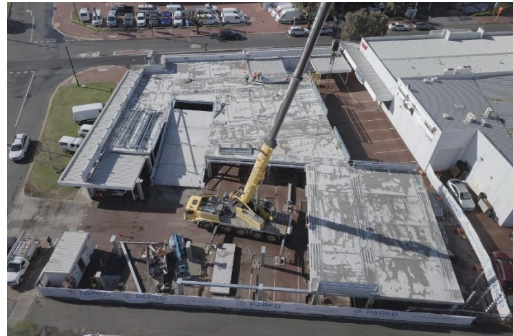
Crane Day 6. Slab panel installation complete
