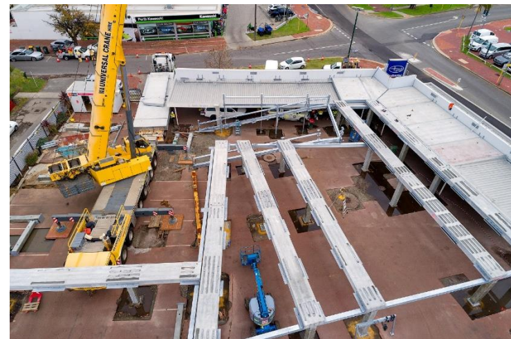
Crane Day 4. Slab panel installation
