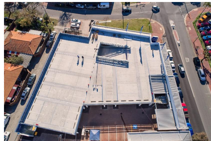
Crane Day 12. Substantial completion of structure
