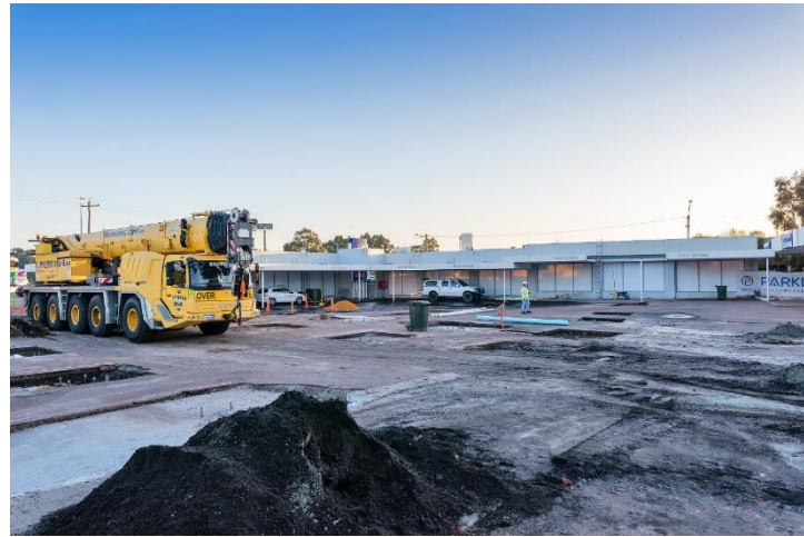
Footings complete and site prepared for PARKD System assembly
