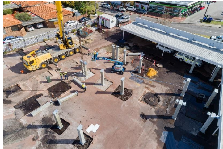
Crane Day 1. Column installation
