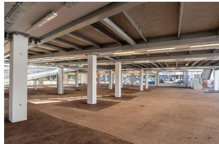
View of underside of the car park structure at Practical Completion
